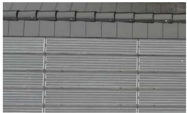
Step 8. Complete the roof space with tiles in perimeter
