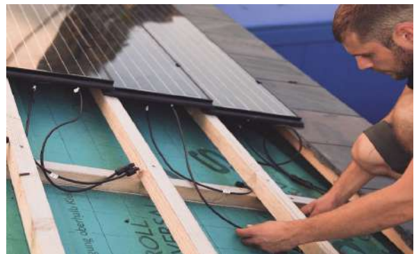
Step 6. Connect the panels to the top of the column
