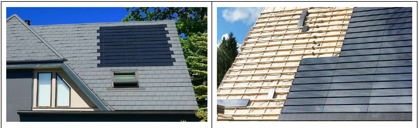
Image 1. Broken Bond vs Straight Column design
