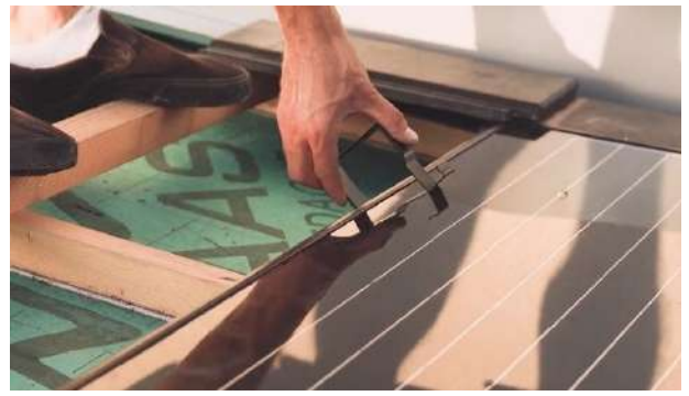
Step 2. Place first panel and attach fittings
