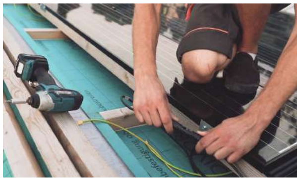
Step 7. Complete string testing, connect last field cable and grounding wire.
