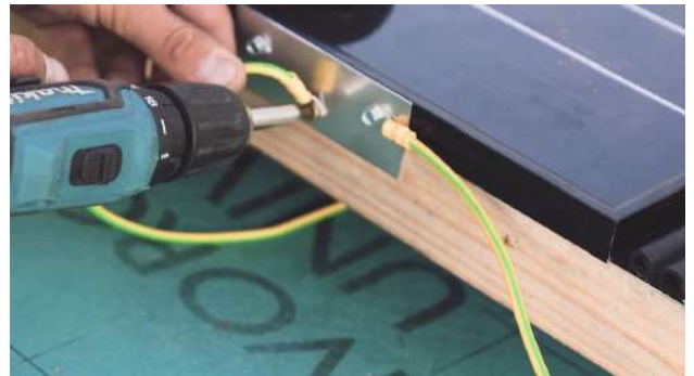
Step 4. Fasten screw on the right with grounding wire
