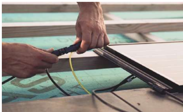
Step 5. Connect the field cable with first panel
